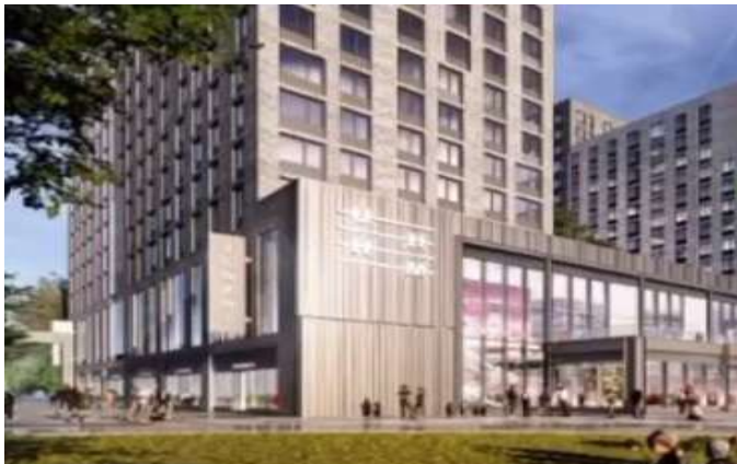
Hip Hop Museum, currently under construction
